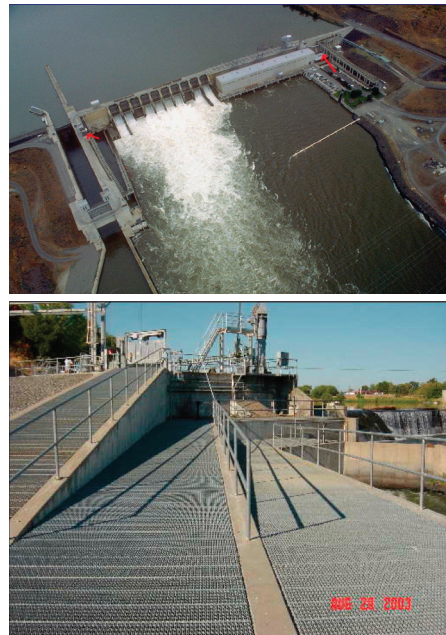
Figure 1. Prosser Dam on the Yakima River in Prosser, Washington (top), and its fish ladder (bottom).
