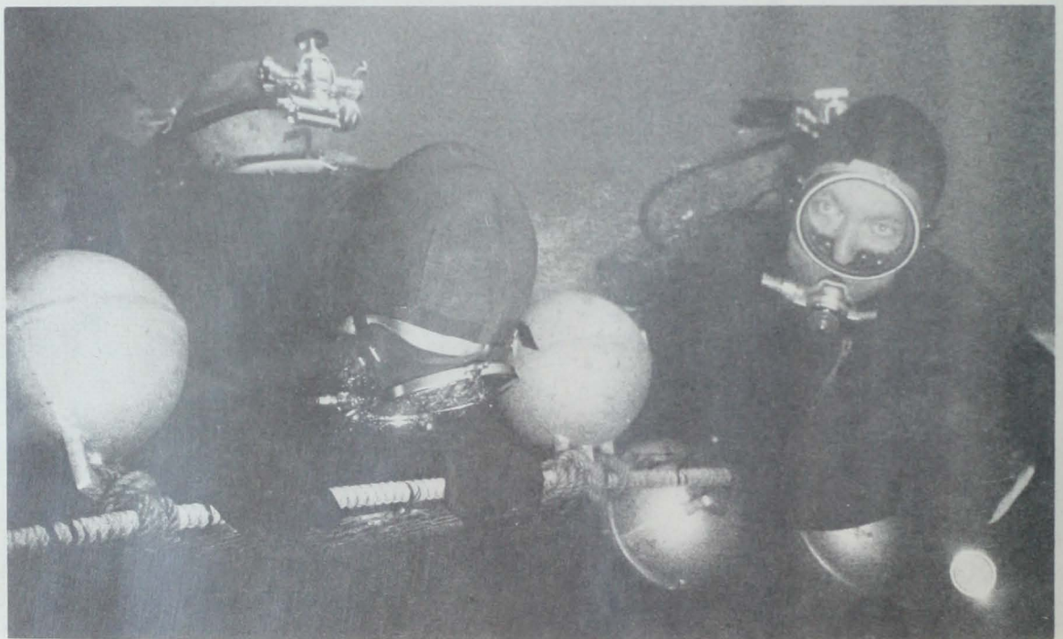
Fig. 5 - Scientists Larry D. Lusz and Ian E. Ellis hang onto headrope of a commercial bottom trawl to visually assess trawl's performance and to observe behavior of fish near the net. (William L. High)
