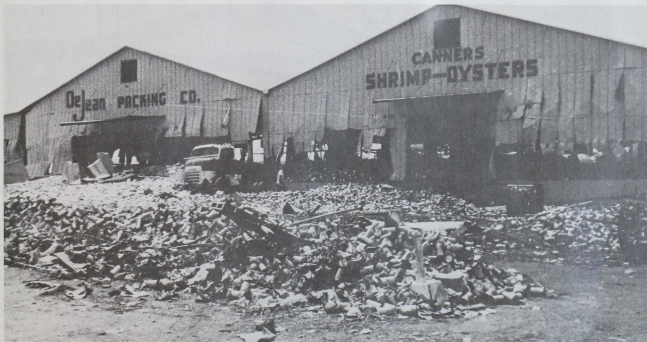
Fig. 2 - Some of 200,000 damaged cases of canned seafood in Biloxi.
