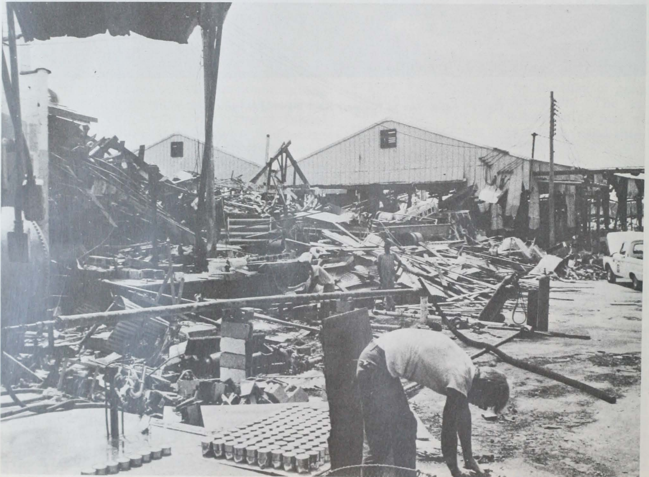
Fig. 3 - Cleanup begins in Biloxi.
