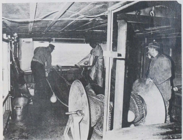
Fig. 8 - Hydraulic powered net reel used to retrieve and store trawl net.
