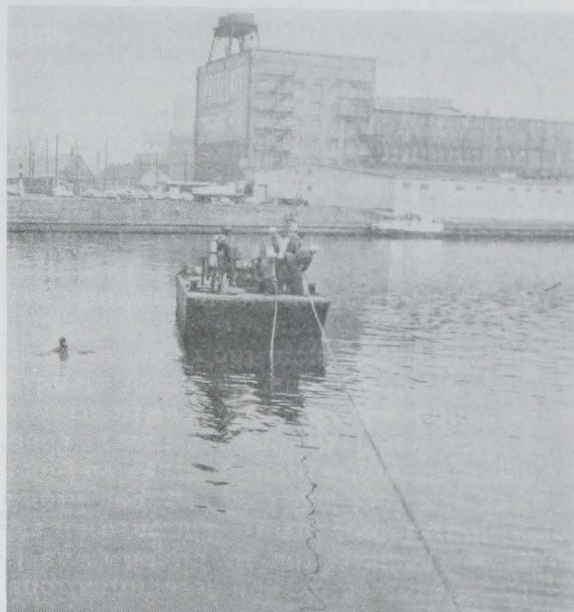
Fig. 4 - Reeling out hose and chain.
