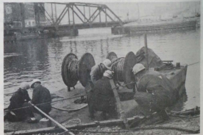
Fig. 3 - Barge used to place air hose.
