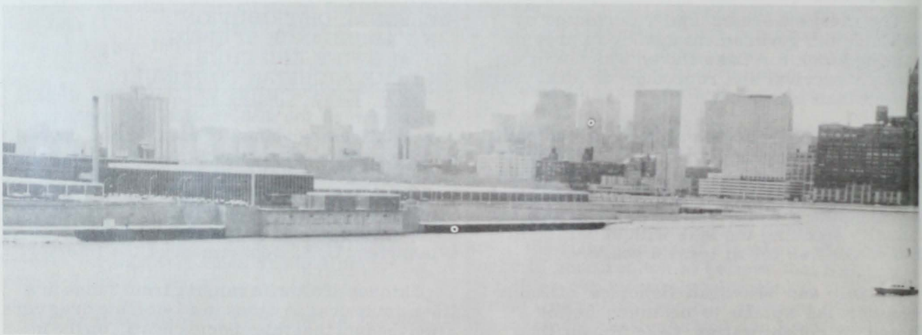
Fig. 2 - Chicago Central District Filtration Plant which supplies water to 2.5 million Chicagoans. Faint white streak near shore at left is the air bubble curtain in operation--used to prevent alewife plugging of water intake screens.
