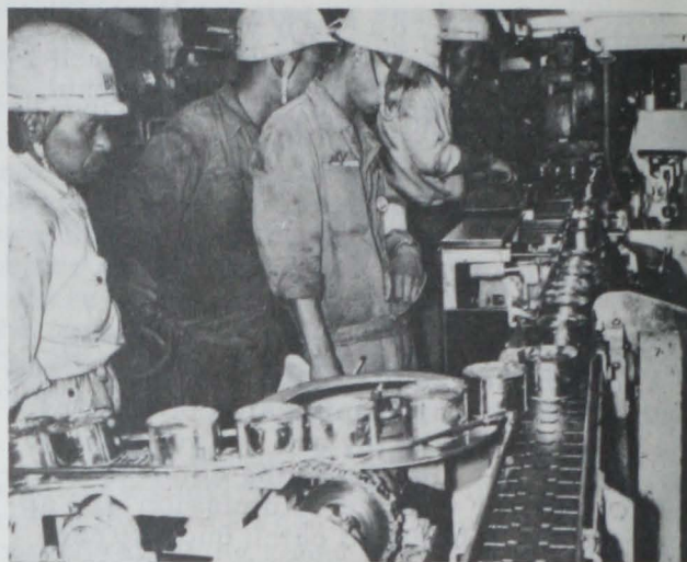
Fig. 5 - Weight checker--cans weighing short are picked out of line by means of a "phototube." Men are timing flow of cans.
