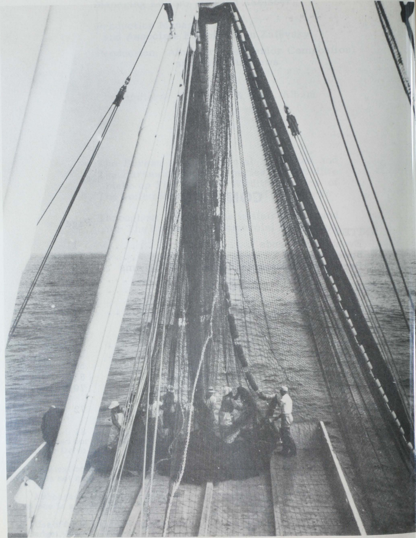
Stacking purse seine net on the tuna clipper "West Point" (BCF Tuna Resources Laboratory, La Jolla, California).
