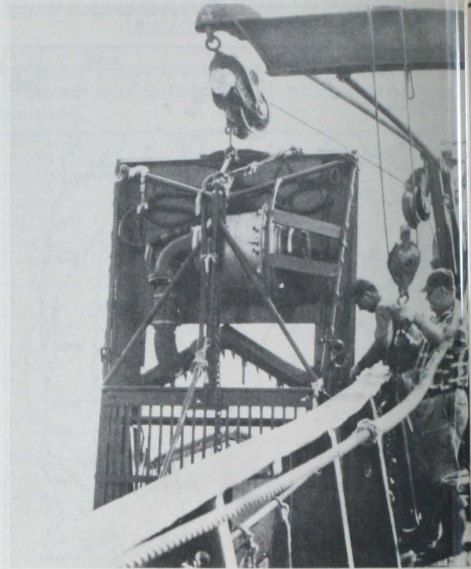
Fig. 2 - Surf clam dredge equipped with electrically-driven 65 horsepower pumping unit.
