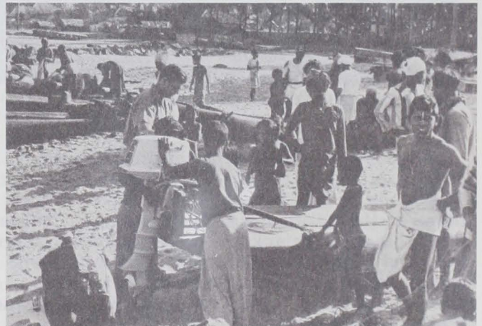
Fig. 1 - An FAO technologist helps Ceylonese fishermen fit an outboard motor to a log raft known as a "teppam."
