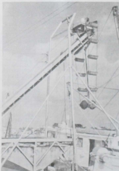
Fig. 2 - Shrimp conveyor unloader at Aransas Pass, Tex.
