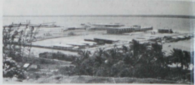
Fig. 1 - Alvarado fishing Port--left to right, boat dock, marine ways and net locker, mooring inlet, offices for fish buyers, ice plant, fish receiving and auction area, fillet lines, processing plants (freezing, canning, salting, smoking, drying), reduction plant for offal.
