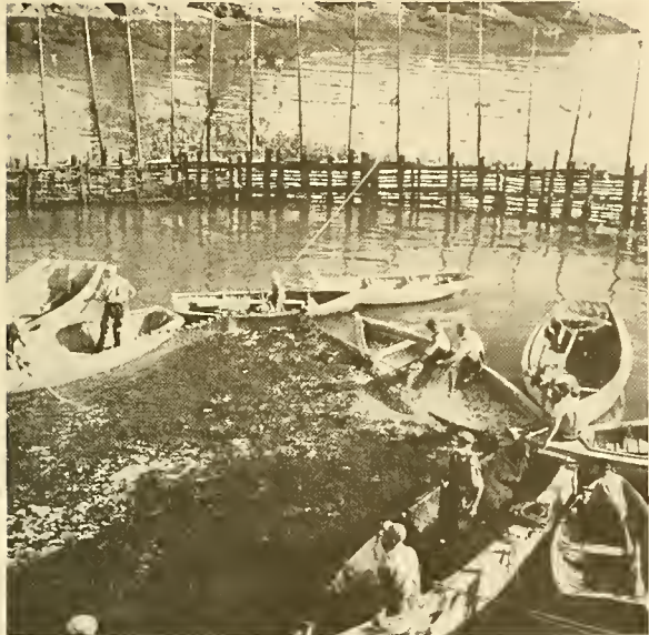
Fig. 2 - "Seining the weir" (concentrating the fish into a mass by gradually decreasing the net space) in a 60-foot sardine weir off the Atlantic Coast.
