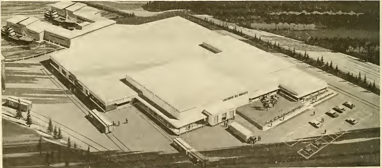
Fig. 4 - New fish-processing plant in Lunenburg, Nova Scotia. Designed to efficiently handle fish by a system of conveyor belts from the vessel unloading pier to the final freezing of the packaged processed fish products. Vessel unloading facilities are completely enclosed.
