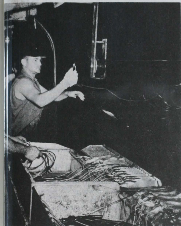
Fig. 2 - Long-line gear on M/V Delaware is set at night from the port-quarter deck. Baited branchlines (5-fathoms) are clipped on the mainline at 20-fathom intervals. Note hinged cover of tub which opens as a bait tray. Hooks and baits (squid and herring) are separated by metal dividers to prevent snarls.
