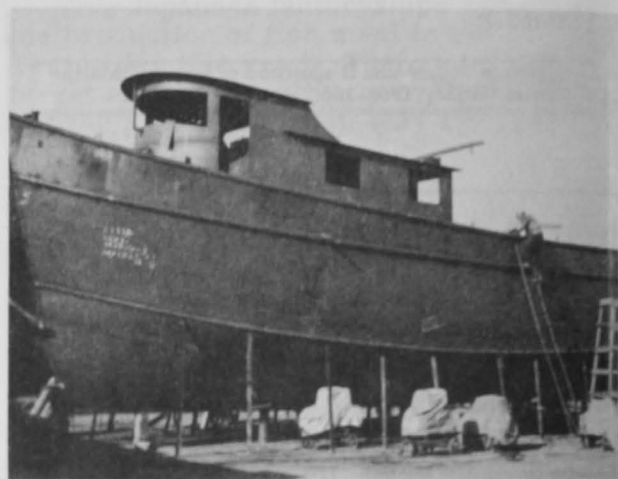
Fig. 1 - Steel shrimp trawler (67 feet) under construction at shipyard in Mazatlan, Mexico, for export to Kuwait.
