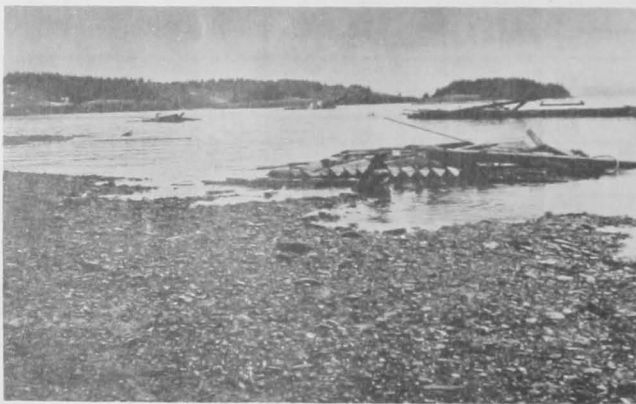
Fig. 1 - This is what the harbor at Kodiak looked like after the earthquake. Pieces of the dock are floating here as well as resting inland. Tides now running 8 feet higher than old maximums.
