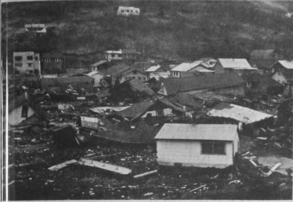
22 - Viewing upper downtown section of Kodiak from a hillside. About 24 dwellings were demolished, and many others were moved as much as 4 blocks off their foundations. A good portion of the business district sustained substantial damage.
