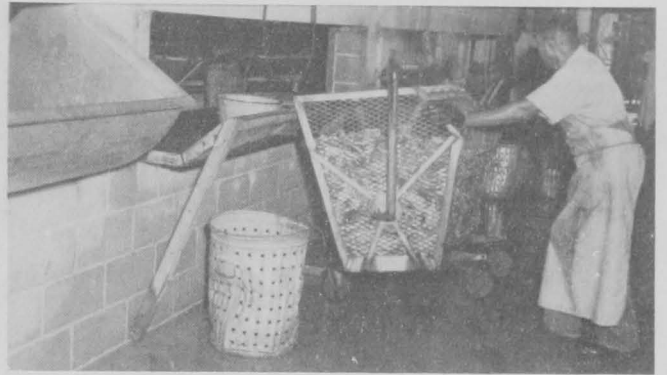
Fig. 14 - Many Gulf Coast plants deback the crabs as soon as they are cool. Here a hoist is lifting a basket until it can be tipped to dump the crabs onto the debacking table.
