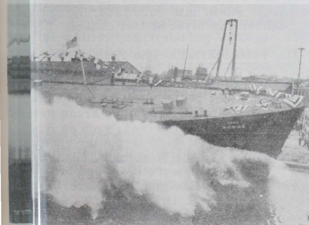
Launching of the Silas Bent at Loraine, Ohio.
