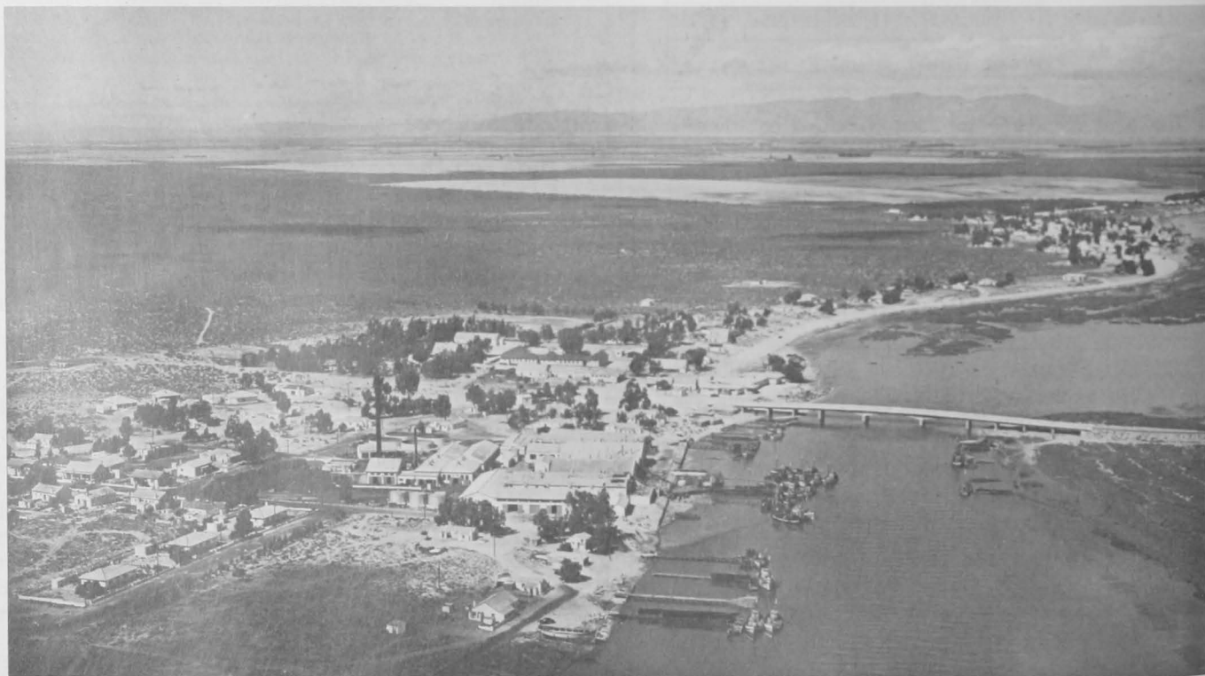
A South African canning and industrial products plant showing mooring jetties.
