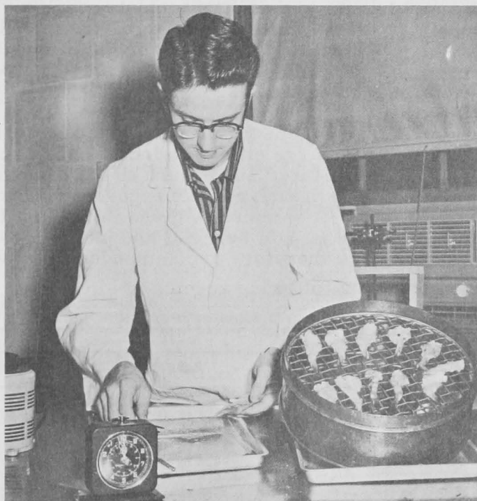
Fig. 4 - The debreaded shrimp are drained on an inclined screen. The operator is picking particles of shrimp meat from the removed material, this operation is not normally required as the amounts of separated flesh rarely is enough to weigh on a gram scale.
