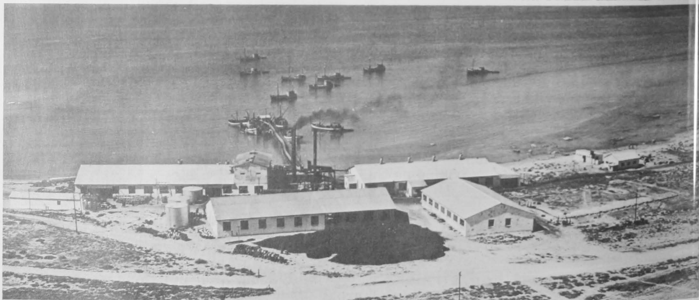
A Cape west coast pilchard and maasbanker cannery and fish reduction plant.
