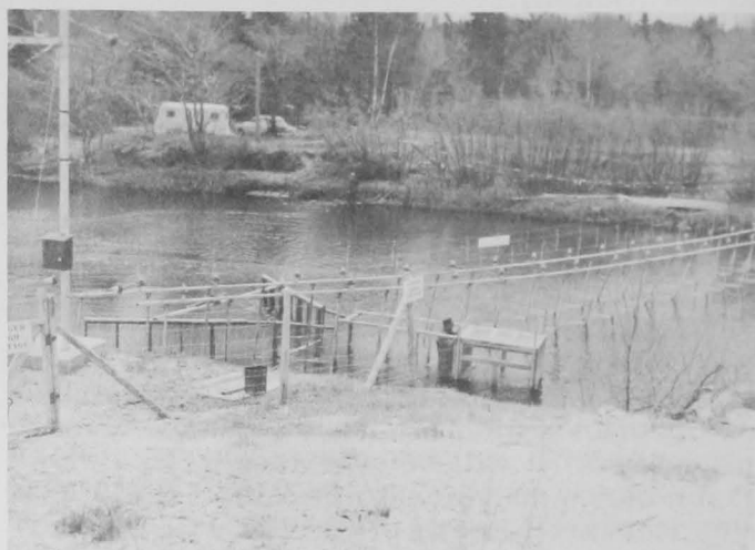
Electric barriers control sea lamprey spawning.
