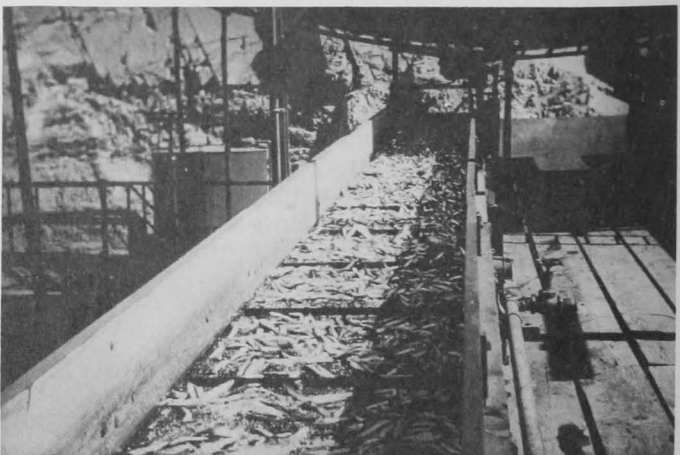
Fig. 3 - Conveyor belt carrying anchovies into fish meal plant for processing.
