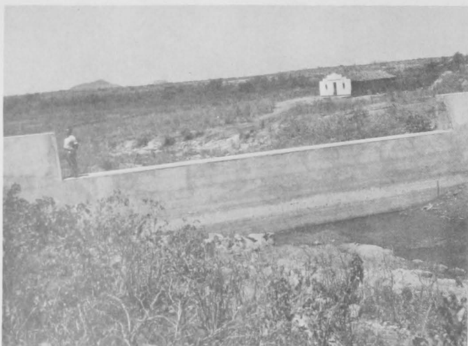
Fig. 12 - "Escama Peixe" (Fish Barrier) built in a drainage ditch to prevent entry of piranhas.
