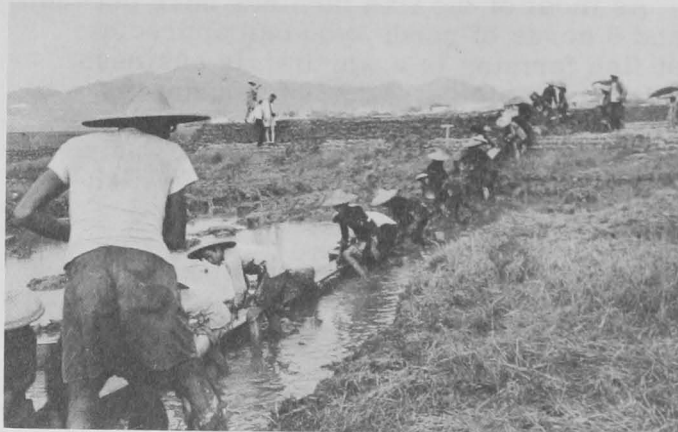
Fig. 1 - How the embankments, causeways and fish ponds are built. Men cut the heavy, greasy clay and women slide it along ramps to be built up into causeways and banks to contain the ponds.
