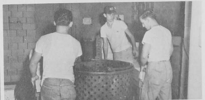
Fig. 41 - The processed cans are removed from the retort basket.
