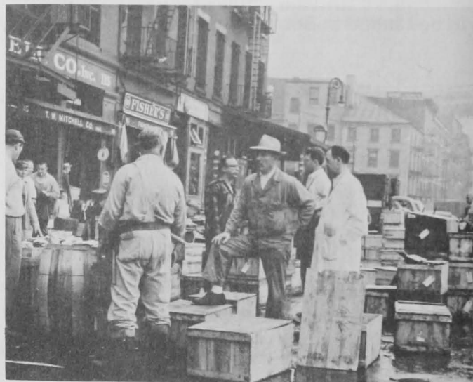
Fig. 2 - View looking north on South Street in the salt-water section of New York City's Fulton Fish Market.
