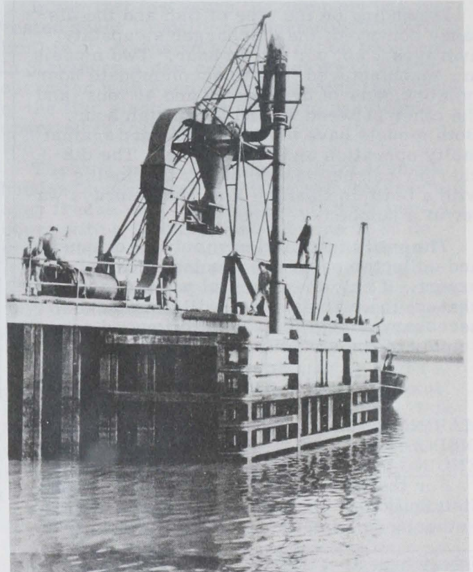
View of air pump for unloading fish from vessels.
