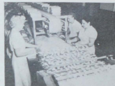
Fig. 39 - All breaded shrimp are hand-packed. Packers line each side of the discharge conveyor from the second breading machine.
