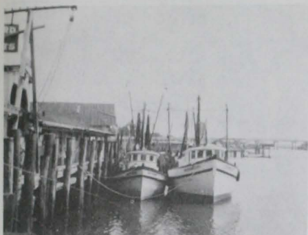
Fig. 3 - Shrimp boats at Thunderbolt, Ga. Note on the left the rope hoist used here, as in most areas, to lift baskets of shrimp from boat hold to dock.
