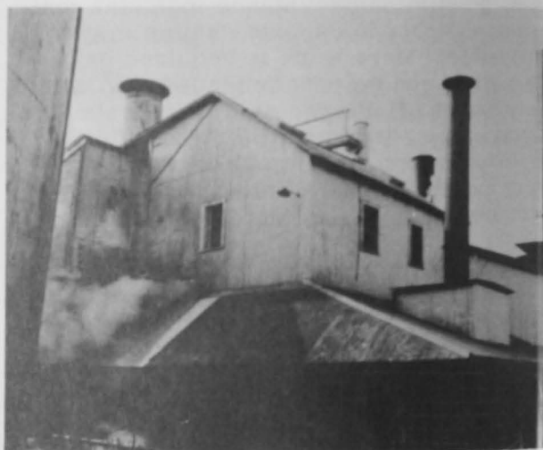
Outside view of a Reedsville, Va., menhaden industrial products plant.
