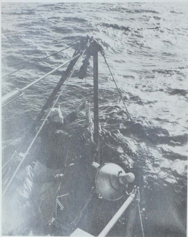
Fig. 2 - Preparing Nansen bottle for lowering to record temperature and test the salinity of sea water.
