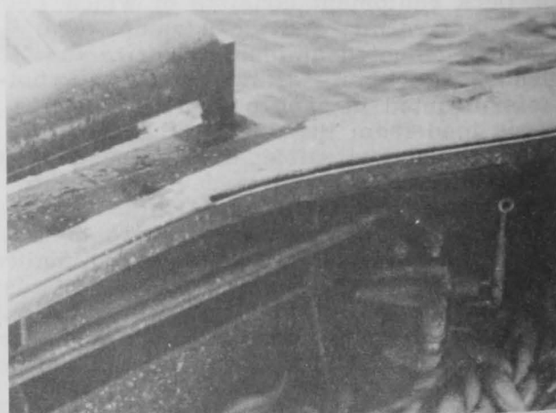
Fig. 5 - Controls for the hydraulic stern ramp rams are located near the stern bulwarks.
