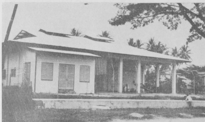
Fig. 16 - Refrigeration unit for cold-storage plant.
