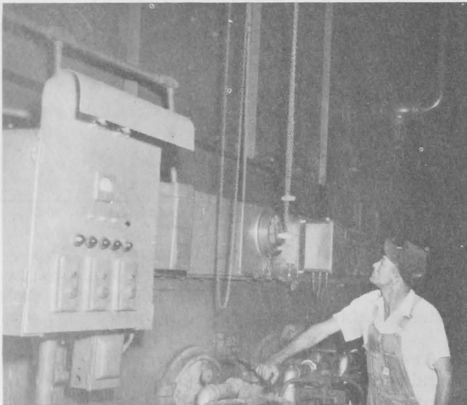
Fig. 1 - Steam power is needed in fishery byproducts plant. It is used to cook the raw fish, evaporate the water in making condensed fish solubles, and in many plants, for heating the meal dryers. This is a scene in a plant at Moss Point, Miss.
