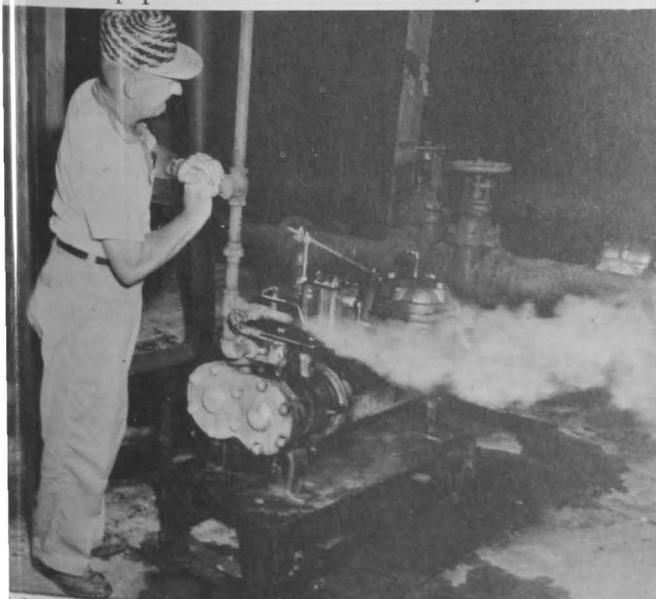
Adjusting valve on a steam pump in the fish solubles unit of a fishery byproducts plant in Empire, La.
