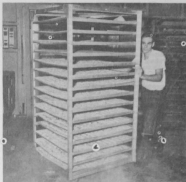
Peeled deveined shrimp laid out individually on large trays. Trays are placed in a roller rack holding 15 trays. Full rack being wheeled into blast freezer for freezing.
