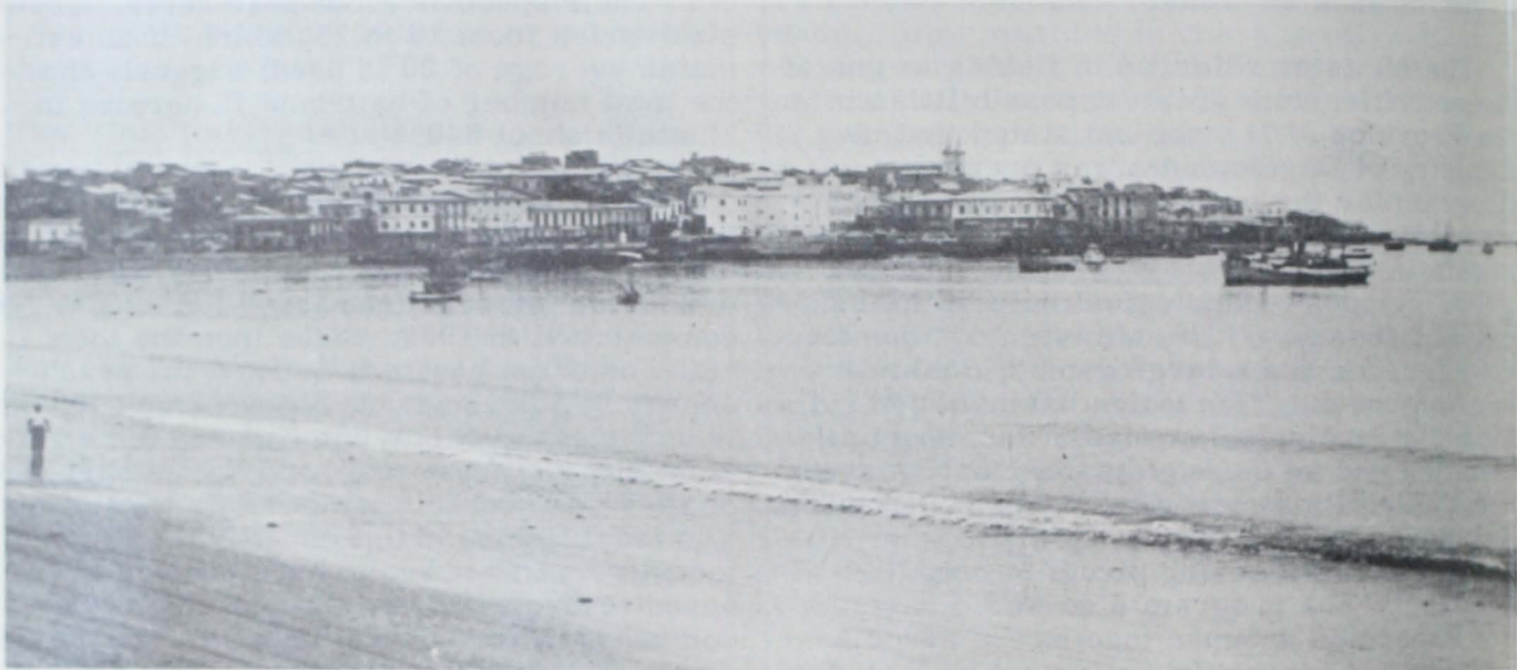
A general view of the Port of Manta.
