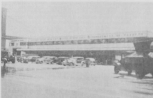
Remodeled Fulton Fish Market completed in 1939.
