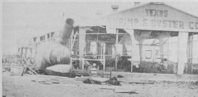
Fig. 3 - Damage inflicted by Hurricane "Carla" to a shrimp and oyster plant at Palacios, Tex.
