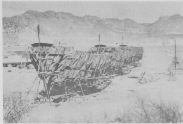
Fig. 3 - Small shipyard near Guaymas, Sonora, Mexico, showing three partially completed 66-foot wooden shrimp vessels.
