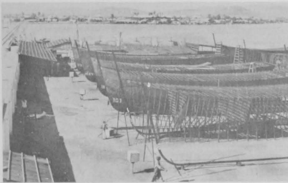
Fig. 2 - Portion of shipyard at Mazatlan devoted to construction of steel vessels.
