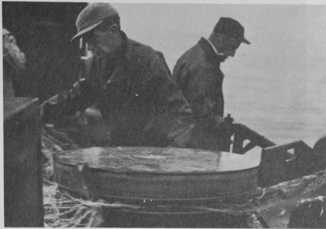
Fig. 3 - Power is supplied to the net-lifter rotor, pictured here, by a small gasoline engine. The fisherman in the foreground is helping to free the gill net from the pawls which grip the net as it comes around the rotor.
