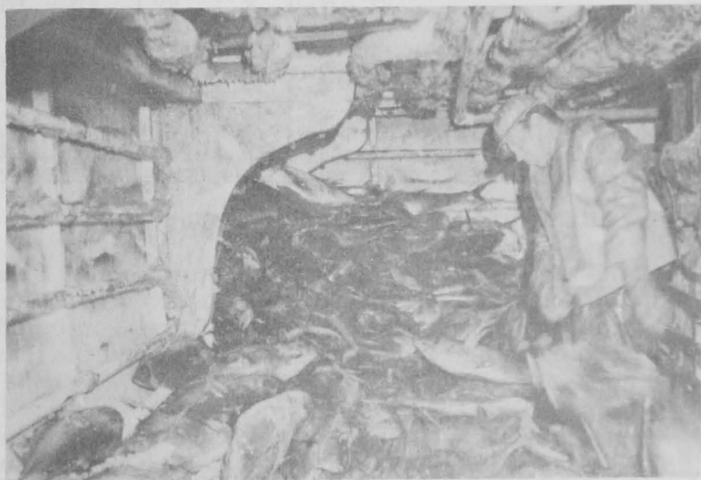
Fig. 6 - Starboard view of the Jo Ann's hold. Notice ice on coils. These coils, as well as those on the sides, are the ones that the water is sprayed onto.
