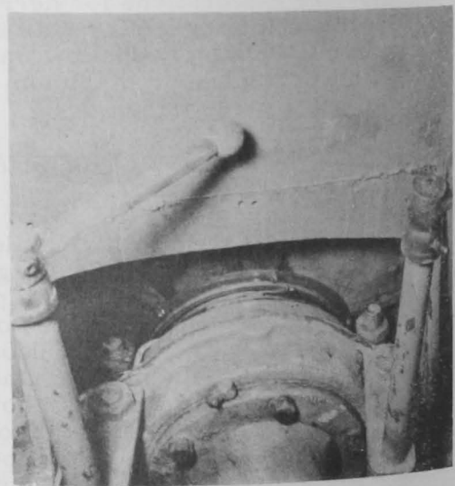
Fig. 7 - Access port of the trawl winch showing location of the slip rings between the winch shaft bearing cap and the drum flanges.
