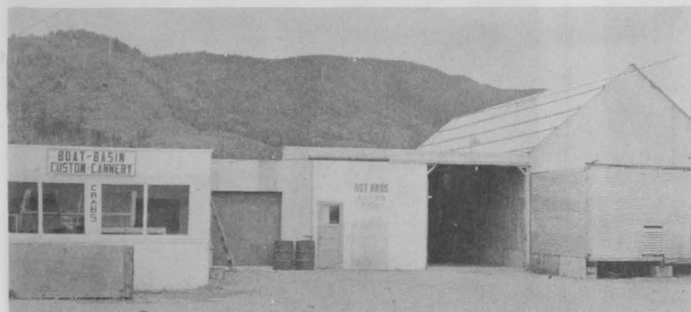
FIG. 6 - ONE OF THE THREE COMMERCIAL FISH-PROCESSING FIRMS LOCATED ON FISHERMAN'S WHARF.
