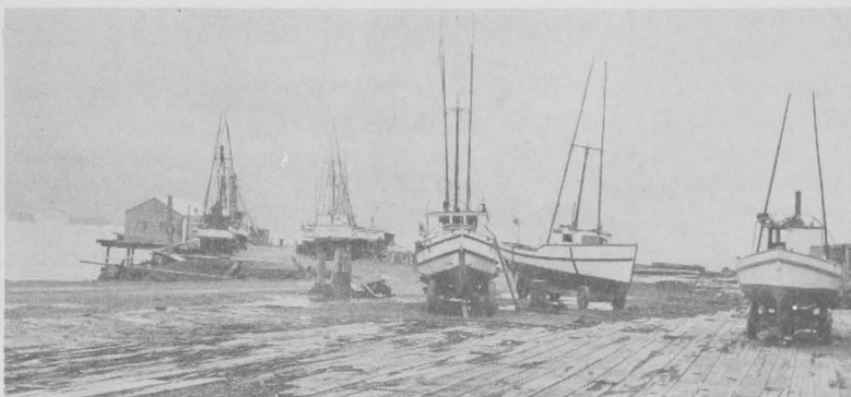
FIG. 4 - TROLLERS ON DOCK. NOTE HOW THE USE OF THE LARGE DOLLIES PERMITS THE TROLLERS TO BE MOVED EASILY TO ANY DESIRED LOCATION. THESE TROLLERS ARE DAY BOATS: THAT IS, THEY LEAVE IN THE MORNING AND RETURN IN THE EVENING OF THE SAME DAY.
