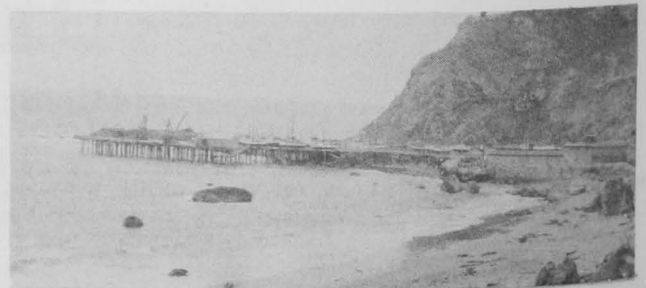
FIG. 2 - THE DOCK. NOTE THE DERRICK USED TO LIFT THE TROLLERS OUT OF THE WATER. THE LARGE BUILDING ON THE RIGHT IS THAT OF A FISH COMPANY.
