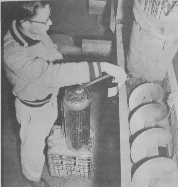
Fig. 3 - Adding oil antioxidant to herring scrap leaving drier.
