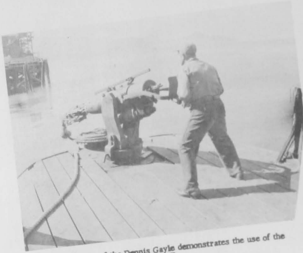
Fig. 13 - Side view of the harpoon gun. Most whales are shot within 80 feet of the vessel. The whale gun is a muzzle loader having a charge of about \frac{1}{2} pound of black powder.
