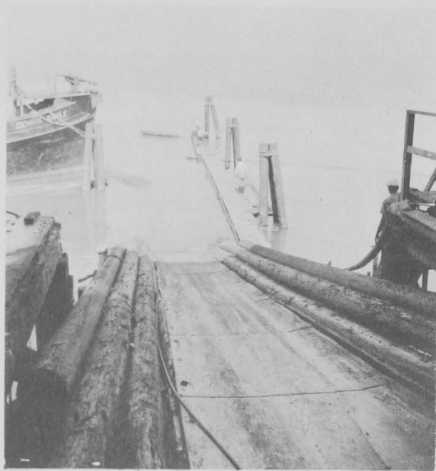
Fig. 20 - Making ready to pull the whale into the station. Note the cable in the foreground. The small rowboat is named the Moby Dick, Jr.
