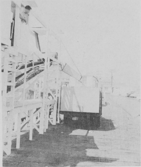
Fig. 5 - Scale house, operator, and tank truck. The operator weighs the anchovies as they come off the elevator. The weighing is done by means of a trip bucket. When the bucket is filled with 500 pounds of anchovies, the operator releases the bottom, and the anchovies then are carried by endless belt to the chute leading into the tank truck.
