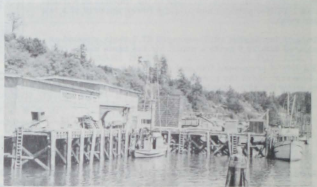
FIG. 2 - DOCK FOR UNLOADING WHOLE FISH.
