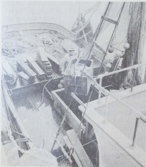
FIG. 3 - UNLOADING FISH FROM DRAGGER. ON THIS PARTICULAR TRIP, ONLY 20,000 POUNDS OF FISH WERE CAUGHT, OWING TO ROUGH WEATHER. THIS VESSEL HAS A 17-FOOT BEAM AND A LENGTH OF 58-FEET. BEING A COMBINATION BOAT, IT CAN BE USED FOR DRAGGING, TROLLING (FOR BOTH SALMON AND TUNA), AND FOR HALIBUT FISHING. NOTE THE DECK HOSE USED FOR CLEANING THE PEN BOARDS. ABSOLUTE CLEANLINESS IS ESSENTIAL TO THE DELIVERY OF QUALITY FISH.
