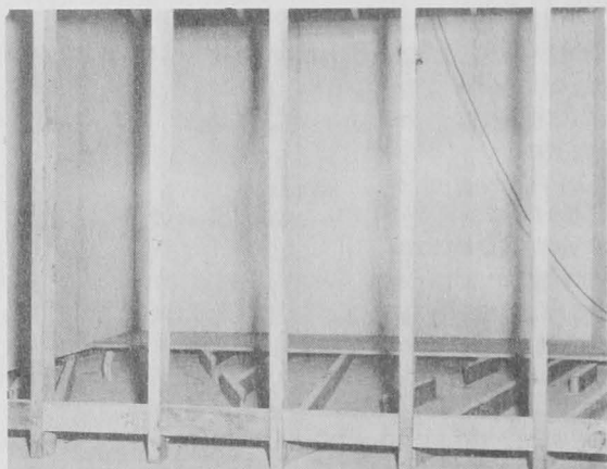
Fig. 1 - Arrangement of air ducts in the floor of the jacketed cold-storage room.
