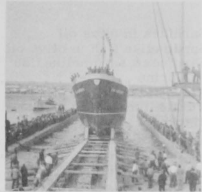
Launching of one of the new trawlers constructed in Portugal.
