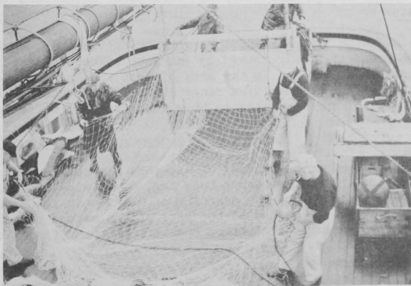
FIG. 3 - CLEARING AND STOWING THE NYLON GILL NET ABOARD THE JOHN N. COBB . THE NET IS SET FROM THE STERN BIN WHILE THE VESSEL MOVES AHEAD SLOWLY.
