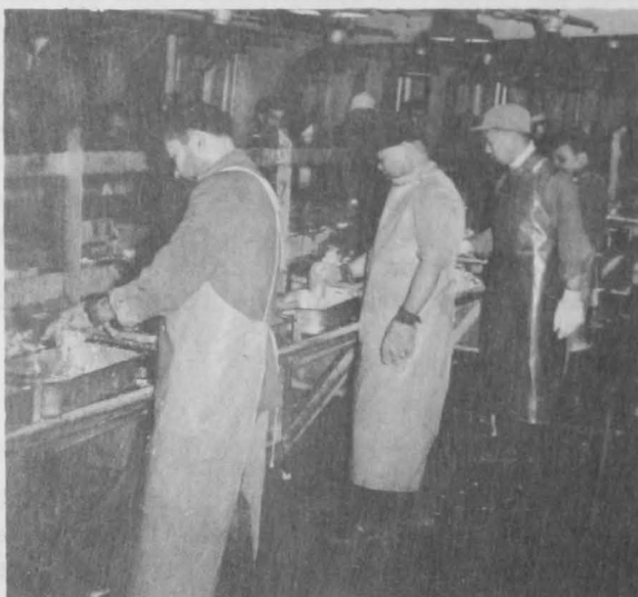
FIG. 2 - THE SHAKING TABLE. THE CRAB MEAT IS REMOVED FROM A LEG SEGMENT BY A QUICK, SHARP RAP OF THE HAND ON A BRACKET COVERED WITH SPONGE RUBBER.
