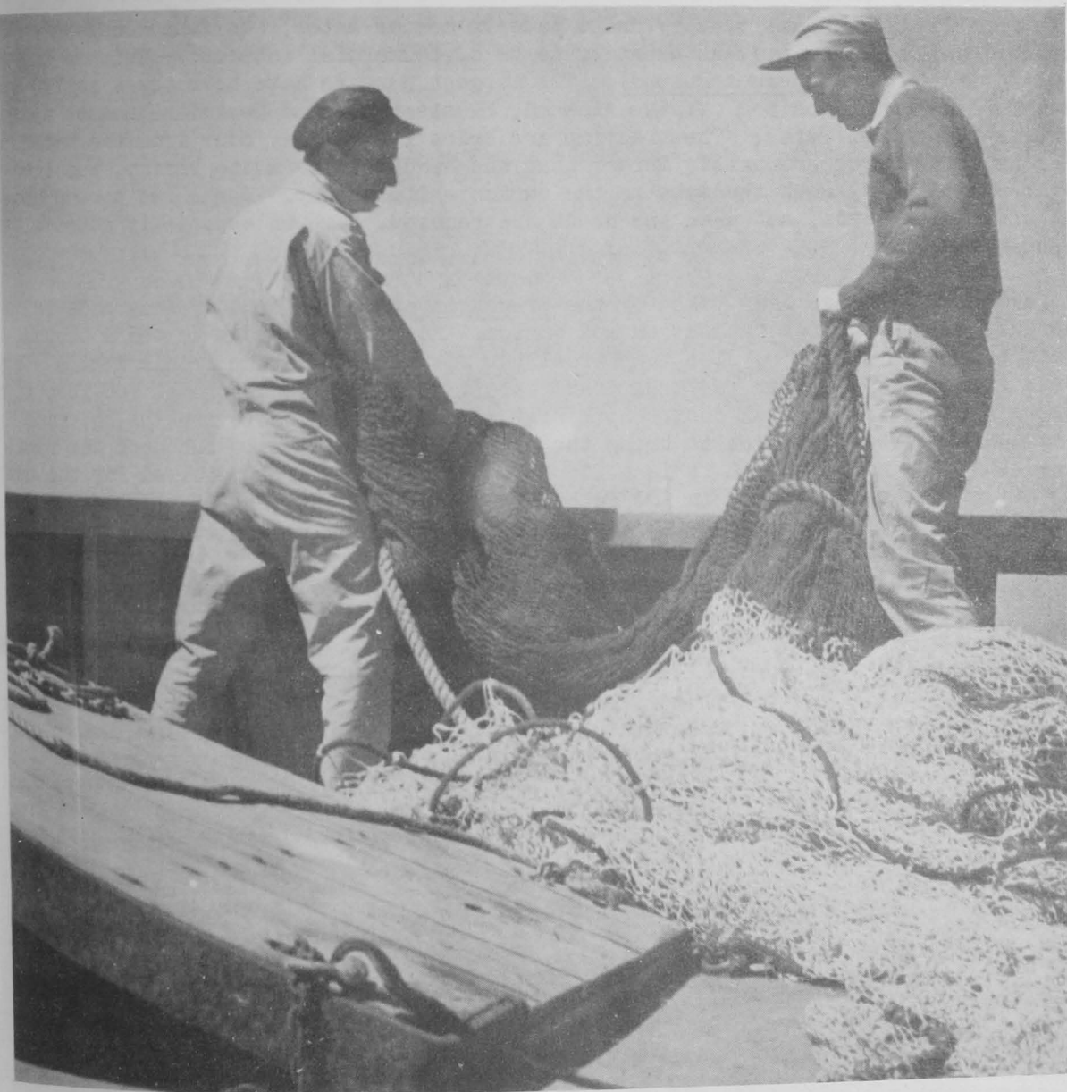
FIGURE 5 - EXPLORATORY FISHING OVER UNKNOWN BOTTOM IS HARD ON GEAR. THIS NET HAS JUST BEEN REPAIRED AT SEA AND IS BEING READIED FOR USE. NEW WEB THAT HAS BEEN PUT IN IS WHITE AND UNTREATED. ONE OF THE LONG-RANGE OBJECTIVES IN THE EXPLORATIONS OF THE OREGON IS TO CHART BOTTOM THAT IS TRAWLABLE.
