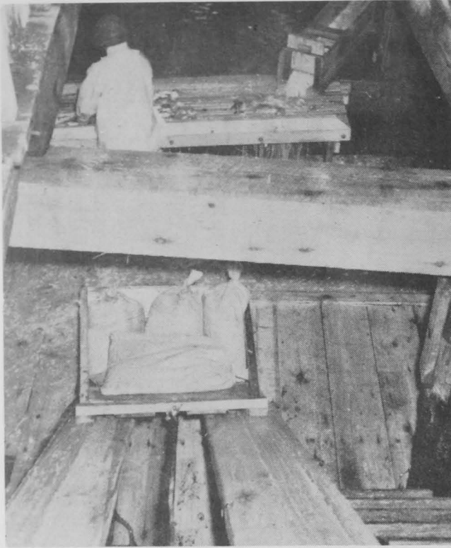
FIG. 6 - THE SACKS OF VISCERA ARE LOADED ONTO THE ELEVATOR AND ARE HAND-WINCHED FROM THE PLATFORM UP TO THE DOCK LEVEL.
